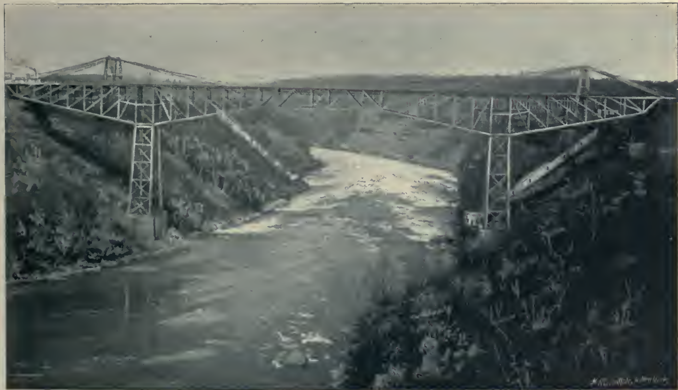
THE CANTILEVER BRIDGE OF THE MICHIGAN CENTRAL.
