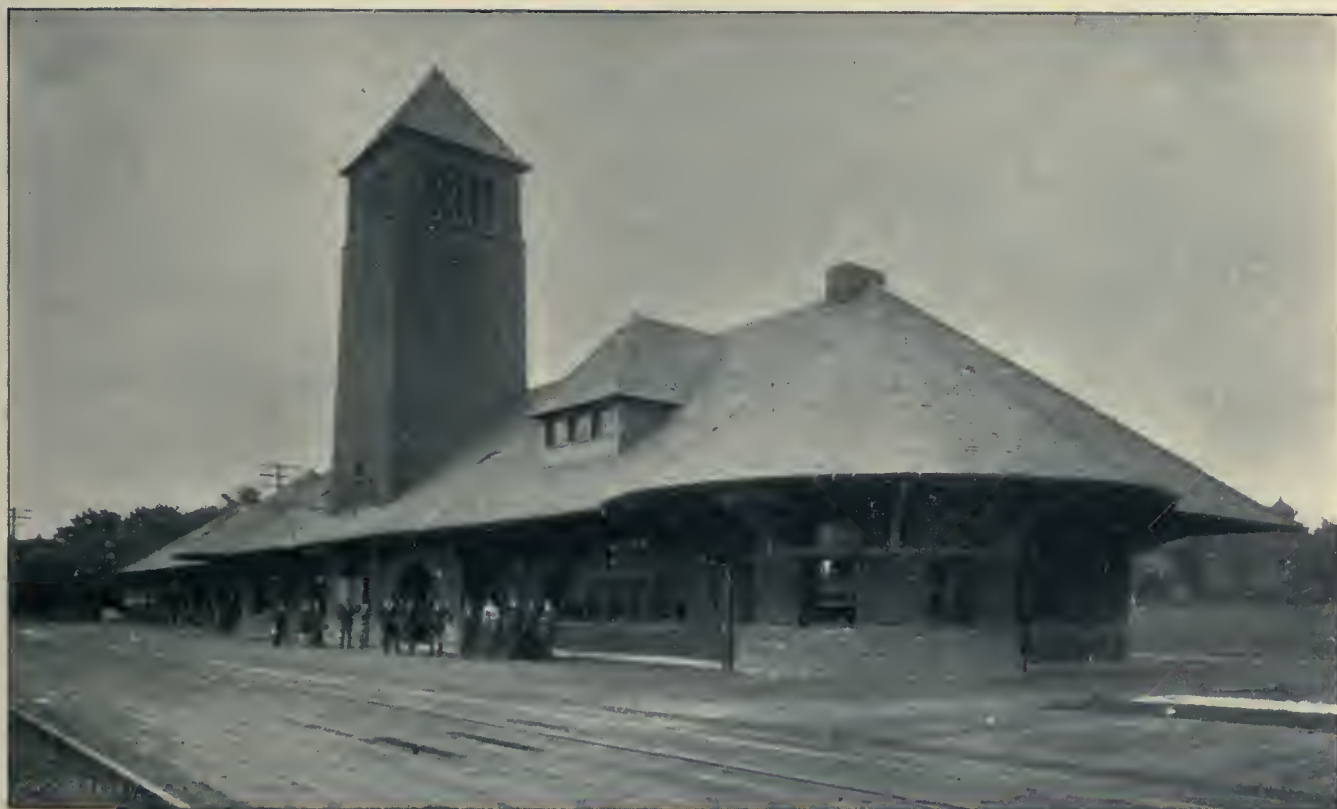
MICHIGAN CENTRAL RAILROAD STATION AT BATTLE CREEK.
